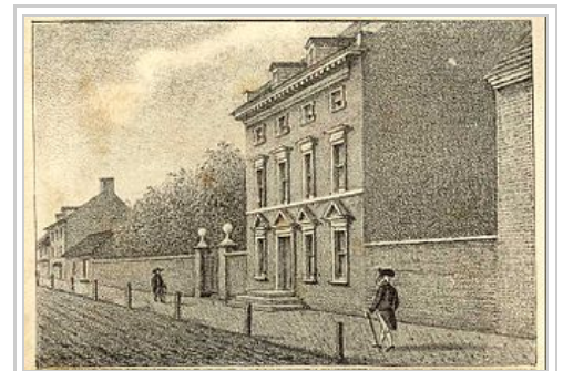
President's House, Philadelphia. The presidential mansion of George Washington before him, Adams occupied this Philadelphia mansion from March 1797 to May 1800. He then became the first President to occupy the Executive mansion in Washington, D.C.
