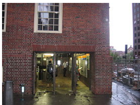
Devonshire Street entrance to State subway station
