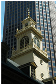
The tower a year prior to restoration, c. 2007
