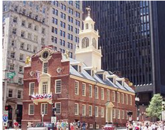
East view of the Old State House, circa July 2003.
