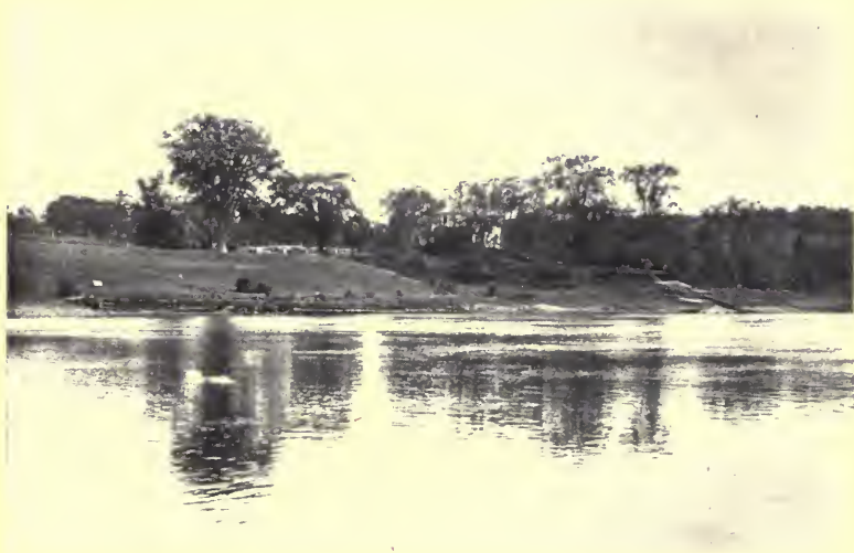
PIPE STAVE LANDING.
