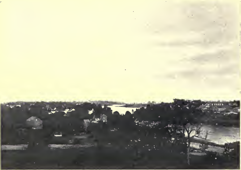
CROOKED LANE, FROM THE ROOF OF THE LIBRARY.
