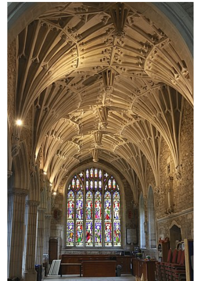
Fan vaulted ceiling of the north aisle ("Dorset Aisle") of Ottery St Mary Church, built by Cecily Bonville, Marchioness of Dorset. She also built the North Porch which displays sculpted Stafford Knots, [31] a heraldic badge of her second husband
